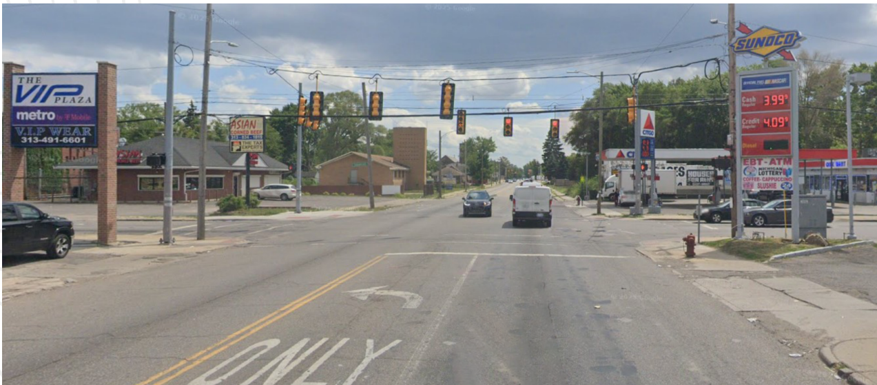
Figure 6.5 The City of Detroit is using SS4A funding to implement several traffic calming measures on Wyoming Avenue, with construction expected to begin in 2026. The above photo shows the existing conditions of Wyoming Avenue.
