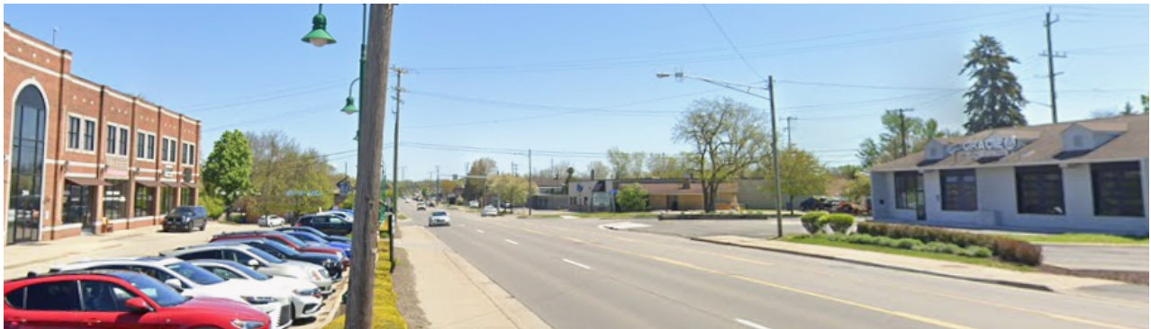
Figure 2.2 While sidewalks currently exist along both Orchard Lake Road and Cass Lake Road, some sections of sidewalk are not buffered from the road or are in need of repair, reducing safety in Keego Harbor's pedestrian environment.
